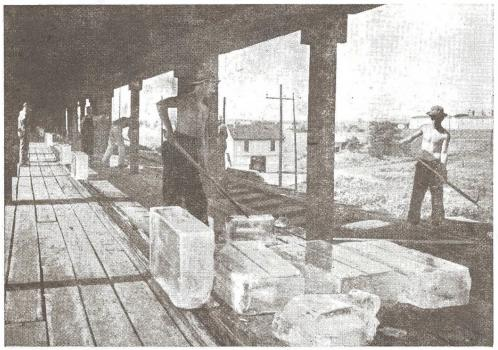
FOUR HUNDRED tons of ice probed from endless conveyor on this platform into refrigerator car bunkers each day make St. Louis Terminal the largest servicer of America's rolling icebox fleet
