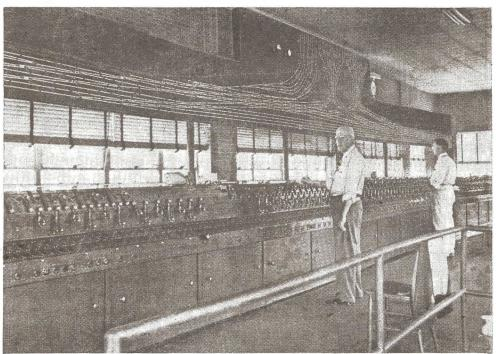
INTERLOCKER PANEL. Levers operate switches and signals for forty-two tracks curving into trainshed
