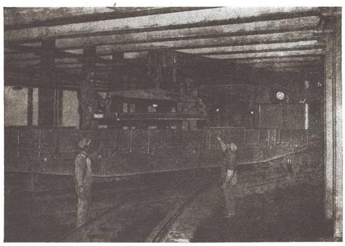
ROADWAY crane clamps its teeth on rail replacement for Broad Street line
